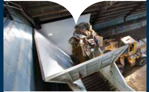
Mixed C&D waste is loaded into the apron feeder for mechanical processing and separation.
